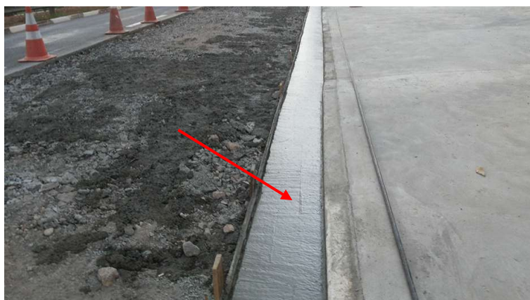
Figura 7: Sarjeta Moldada in Loco
